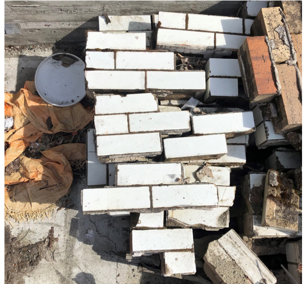
Representative condition of the bricks
