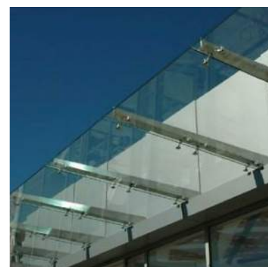
Tempered Glass Canopy / Rain Protection w/ Safety Film, PTD Steel Structure
