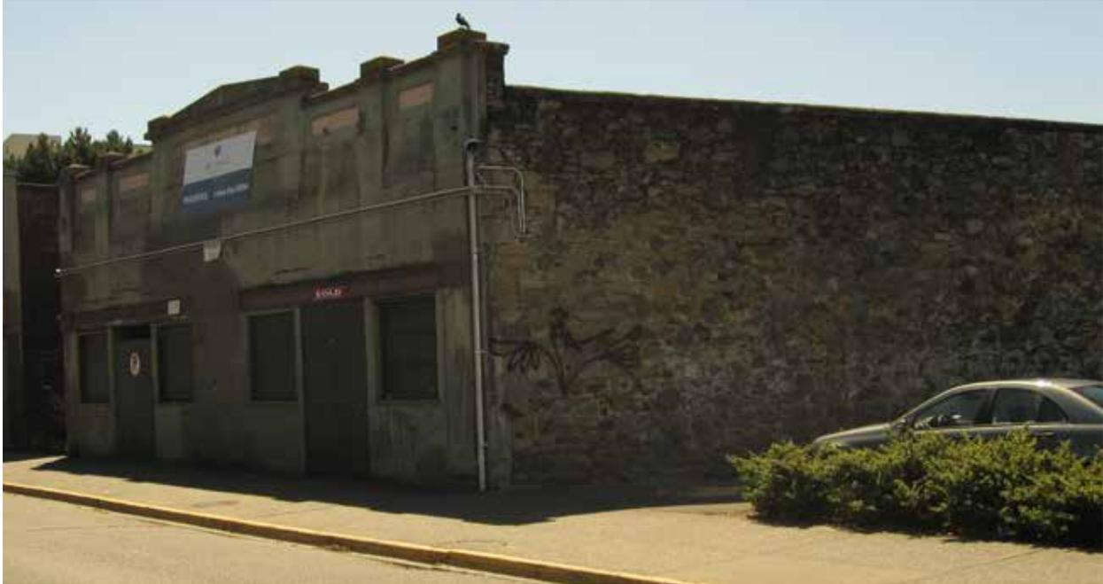
*Current front elevation with late applied stucco of the Fraser Warehouse.*
