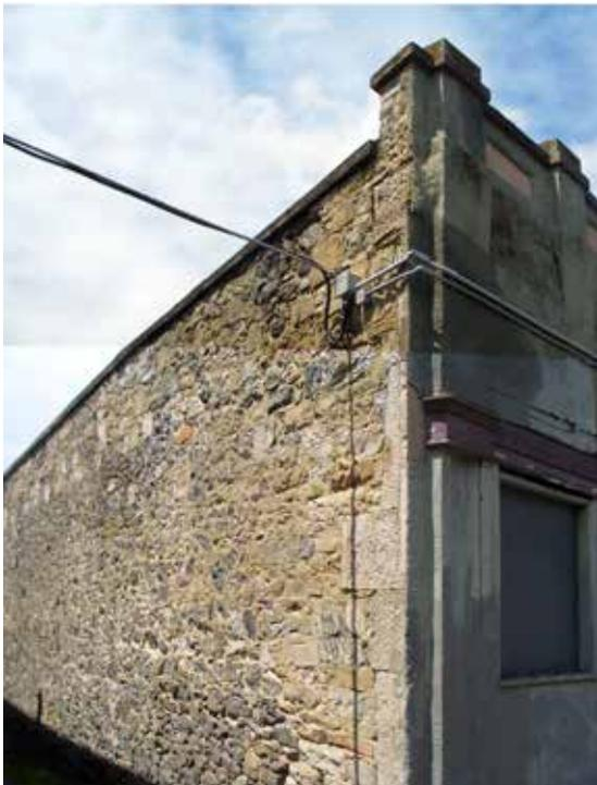
*Current side and front elevations showing the stone construction with quoining on the corner Fraser Warehouse*
