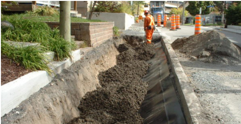
Structural soil installation
