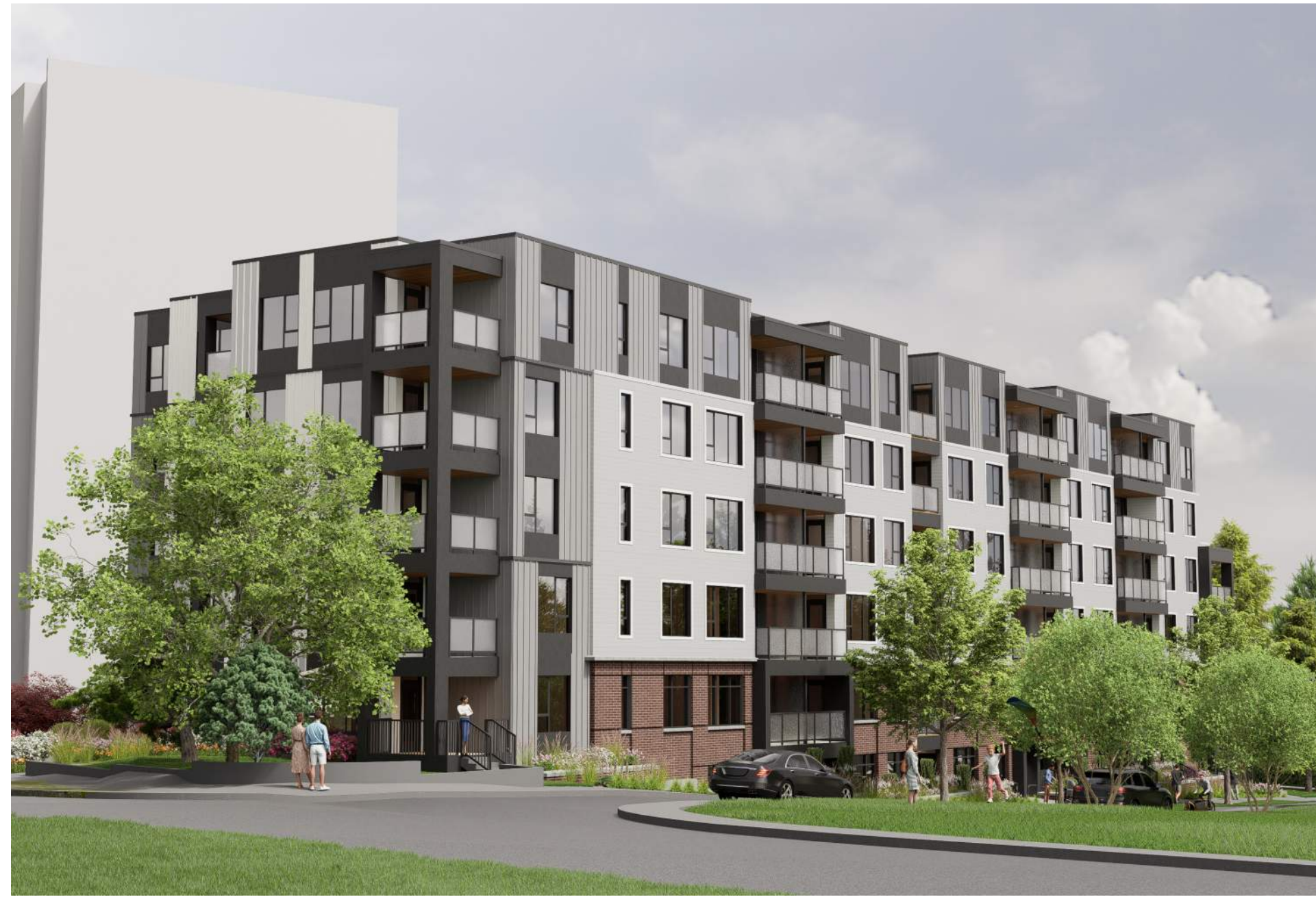
VIEW FROM THE NORTH EAST CORNER AT DOUGLAS STREET AND TORONTO STREET.
