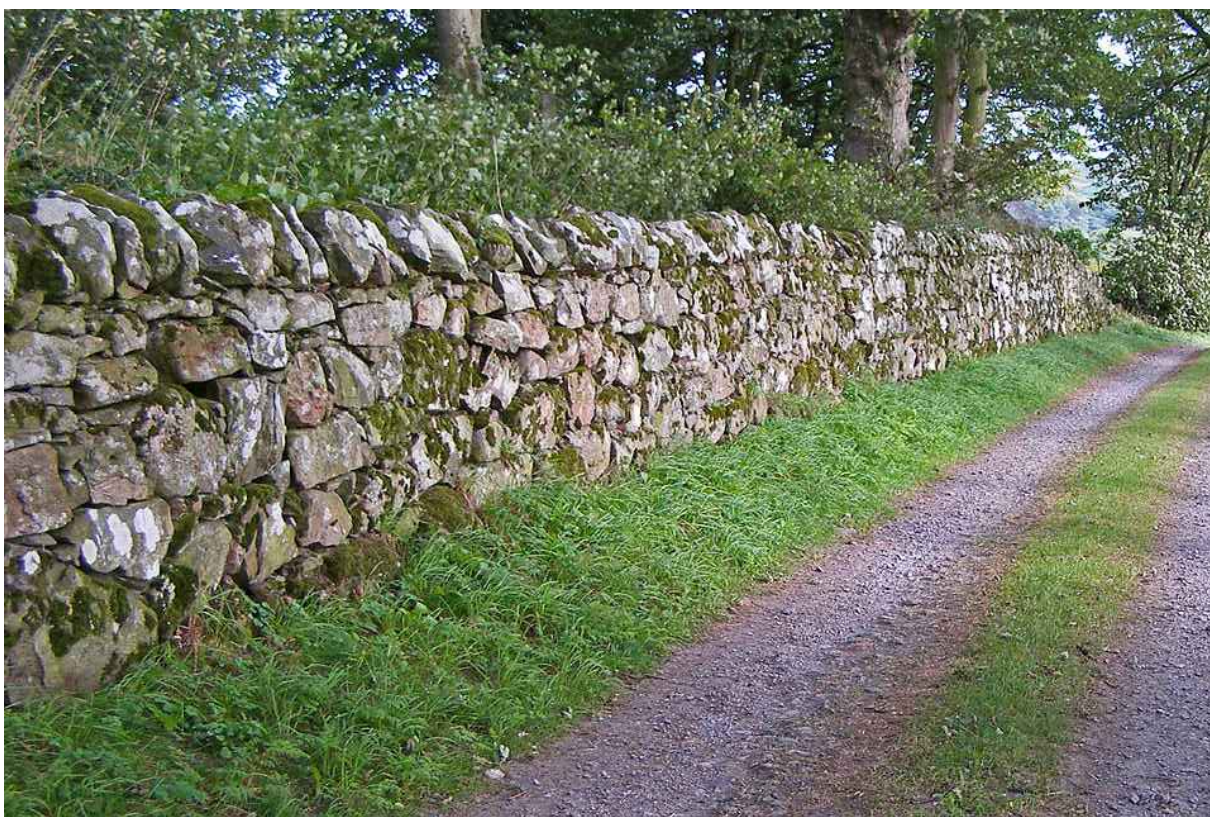
GRANITE STONE WALL PRESERVATION
