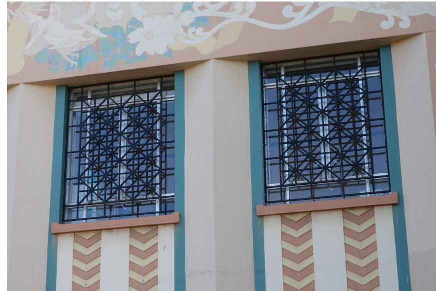
Original metal window screen detail on north elevation
