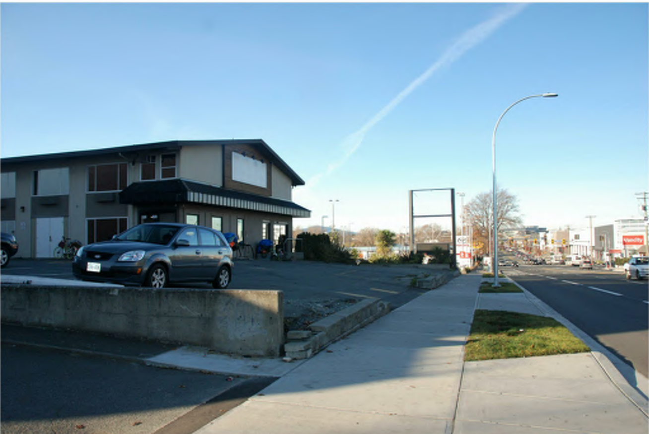
07. Site from Douglas St- looking north
