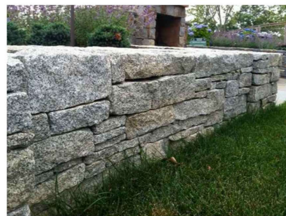
MORTARED HERITAGE STONE ROCK WALL FOR WINDOW WELL RETENTION
