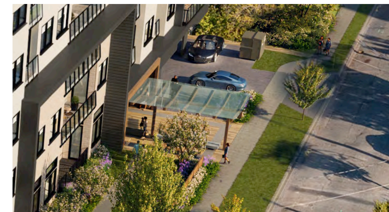
Main Entrance Plaza and Canopy
