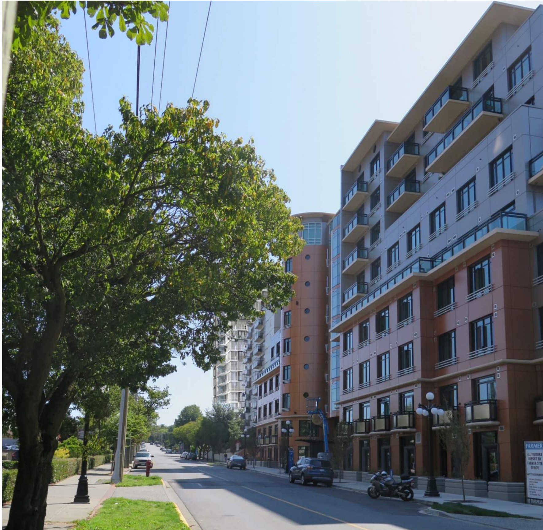
B View Street Looking East
