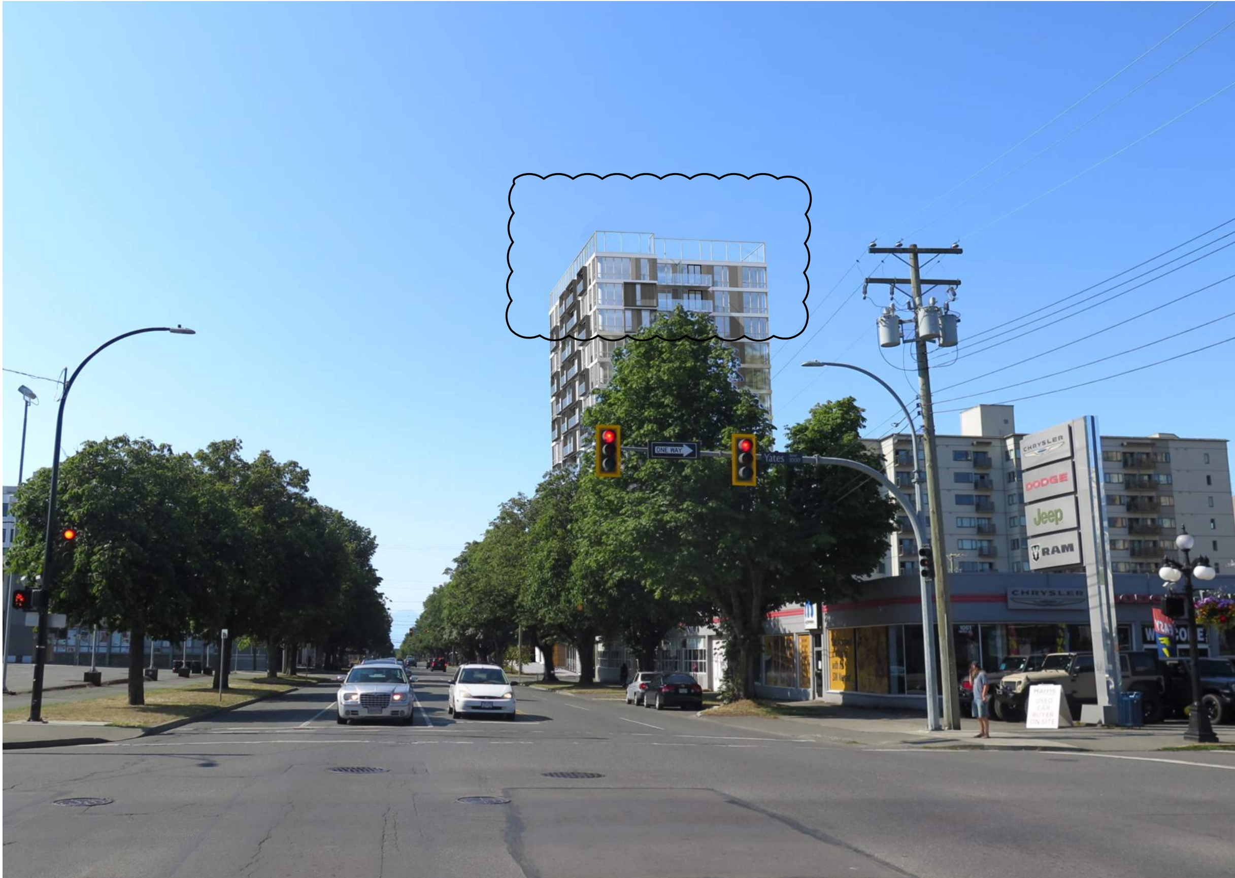
C Cook Street Looking South
