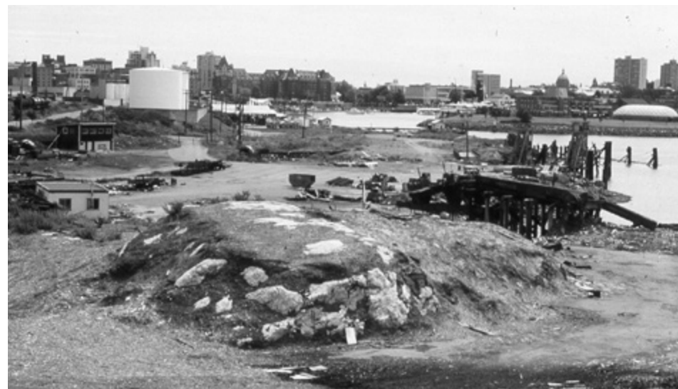
Site looking east, 1983
