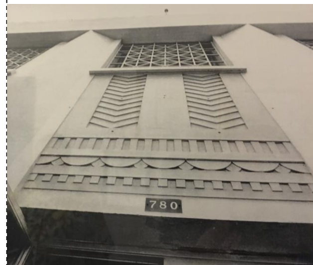
Figure 16: View of chevron spandrels and horizontal bands of vertical beveled geometrics and half-disc motifs, decorative metal window grilles on the north entrance.
