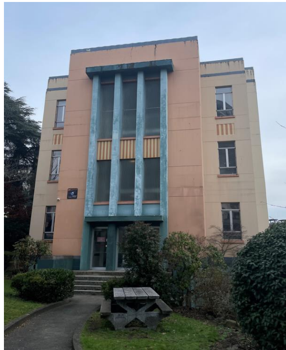
Figure 42: View of west elevation. Vertical pilasters and the closed stair retaining walls to be restored to original appearance clad in marble.
