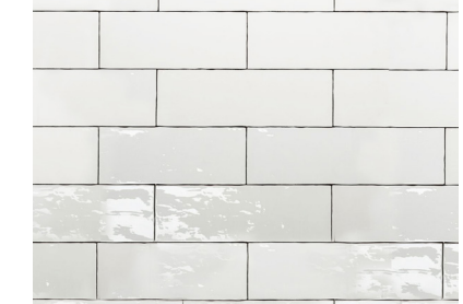
EXISTING WHITE GLAZED BRICK
