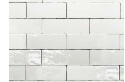
EXISTING WHITE GLAZED BRICK
