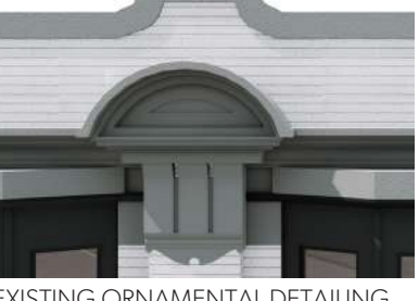
EXISTING ORNAMENTAL DETAILING RESTORED TO HERITAGE COLOUR PALETTE
