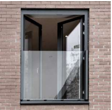
JULIET BALCONIES WITH CLEAR GLASS ON LIVING SPACE WINDOWS FACING FRANKLIN GREEN PARK & HARRIS GREEN PARK
