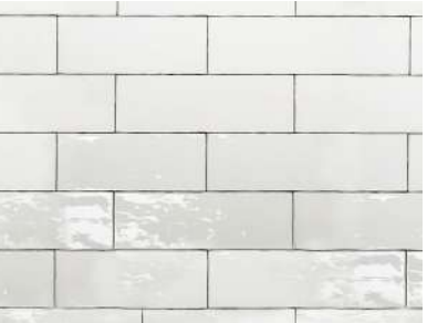
EXISTING WHITE GLAZED BRICK
