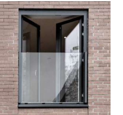
JULIET BALCONIES WITH CLEAR GLASS ON LIVING SPACE WINDOWS FACING FRANKLIN GREEN PARK & HARRIS GREEN PARK
