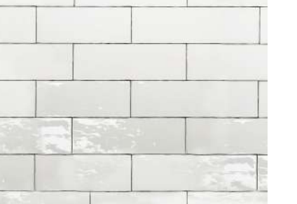
EXISTING WHITE GLAZED BRICK
