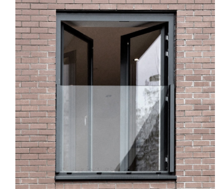
JULIET BALCONIES WITH CLEAR GLASS ON LIVING SPACE WINDOWS FACING FRANKLIN GREEN PARK & HARRIS GREEN PARK
