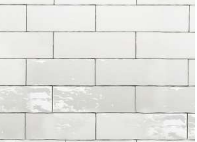
EXISTING WHITE GLAZED BRICK
