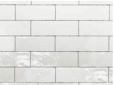
EXISTING WHITE GLAZED BRICK
