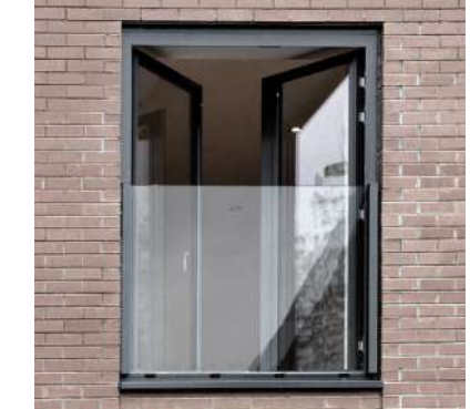
JULIET BALCONIES WITH CLEAR GLASS ON LIVING SPACE WINDOWS FACING FRANKLIN GREEN PARK & HARRIS GREEN PARK
