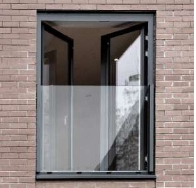
JULIET BALCONIES WITH CLEAR GLASS ON LIVING SPACE WINDOWS FACING FRANKLIN GREEN PARK & HARRIS GREEN PARK
