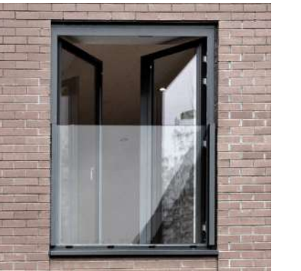
JULIET BALCONIES WITH CLEAR GLASS ON LIVING SPACE WINDOWS FACING FRANKLIN GREEN PARK & HARRIS GREEN PARK
