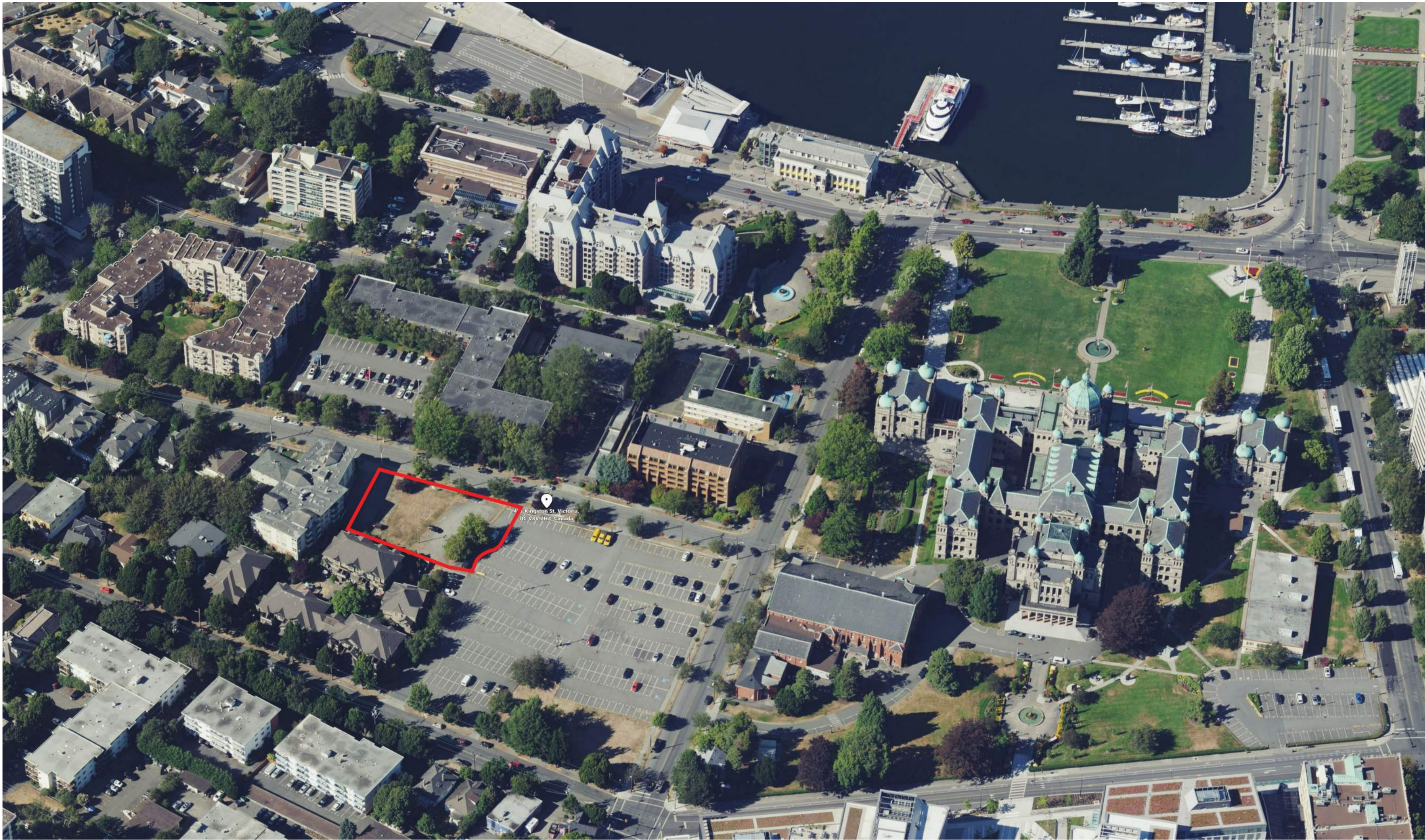
BIRDSEYE VIEW LOOKING NORTHWEST AT EXISTING SITE
