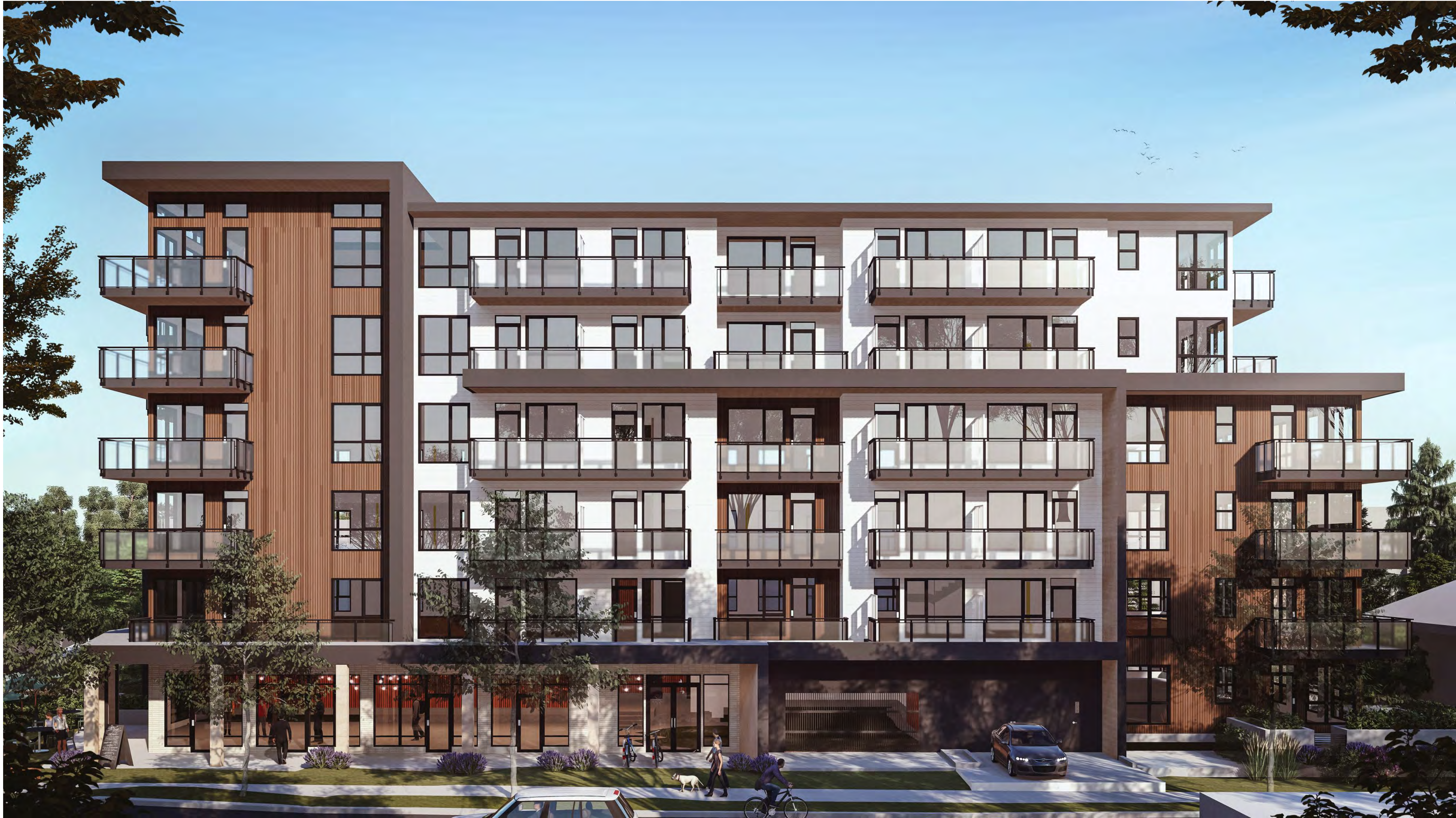
West Elevation - Davie St
