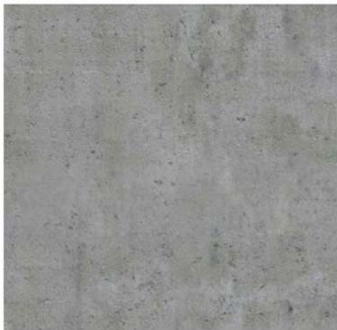
4.1 ▲ EXPOSED CONCRETE FIRE-HALL L1 / SITE
