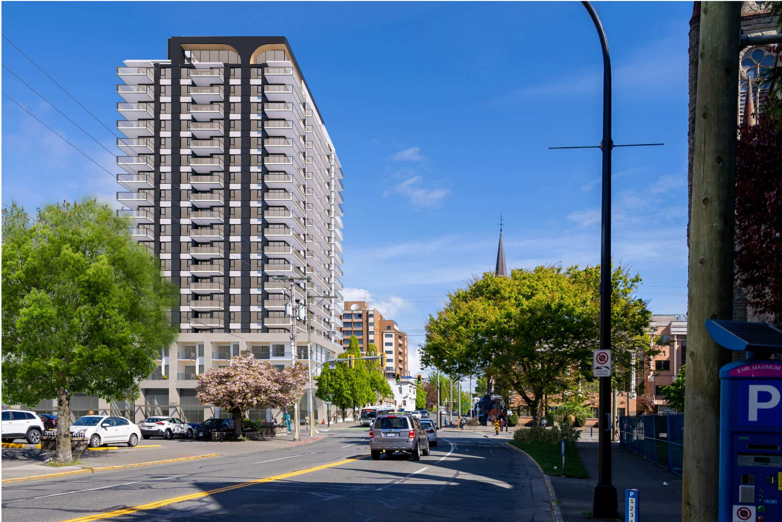
LOOKING NORTH ON QUADRA ST.
