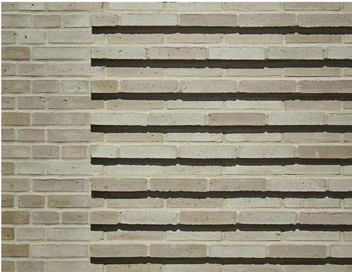
HORIZONTAL BRICK REVEAL DETAILING
