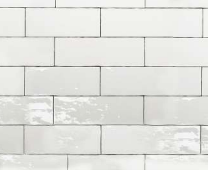
EXISTING WHITE GLAZED BRICK
