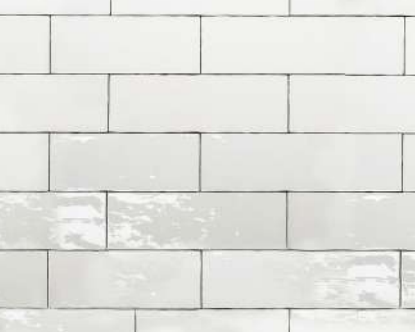
EXISTING WHITE GLAZED BRICK
