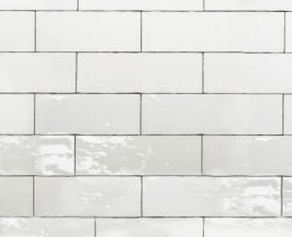
EXISTING WHITE GLAZED BRICK
