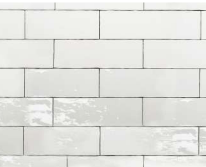
EXISTING WHITE GLAZED BRICK
