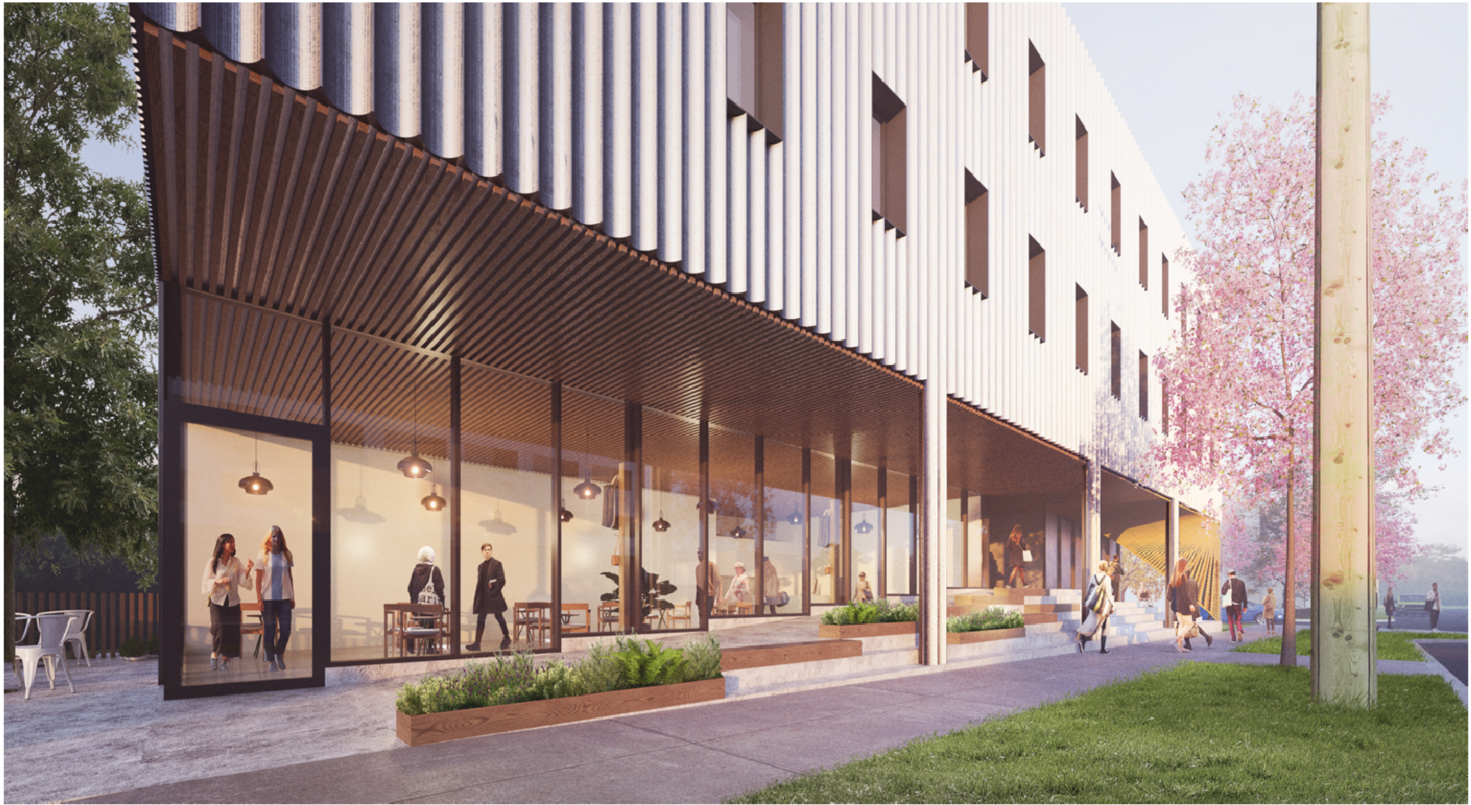
VIEW OF CRU FROM CATHERINE STREET SIDEWALK
