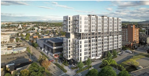
2615-2629 Douglas St. D'Ambrosio Architecture + Urbanism
