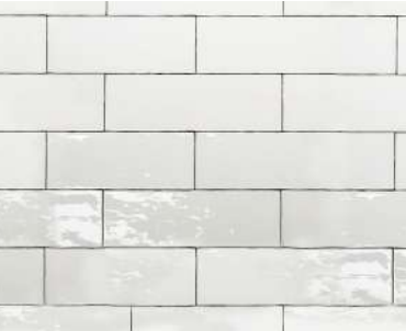
EXISTING WHITE GLAZED BRICK
