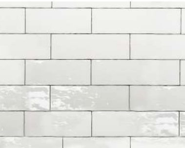
EXISTING WHITE GLAZED BRICK
