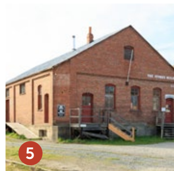
Stores building, view from east (Focus Equities)
