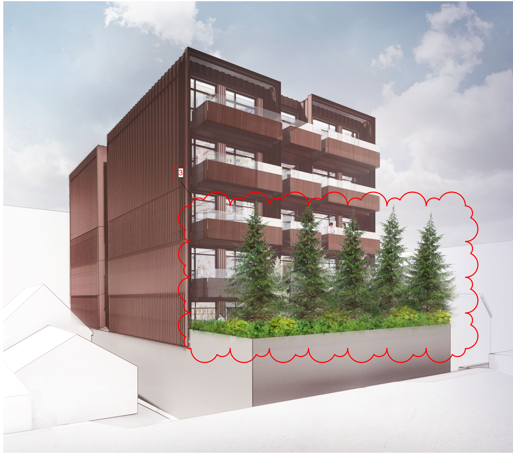
VIEW OF NORTH FACING FACADE
