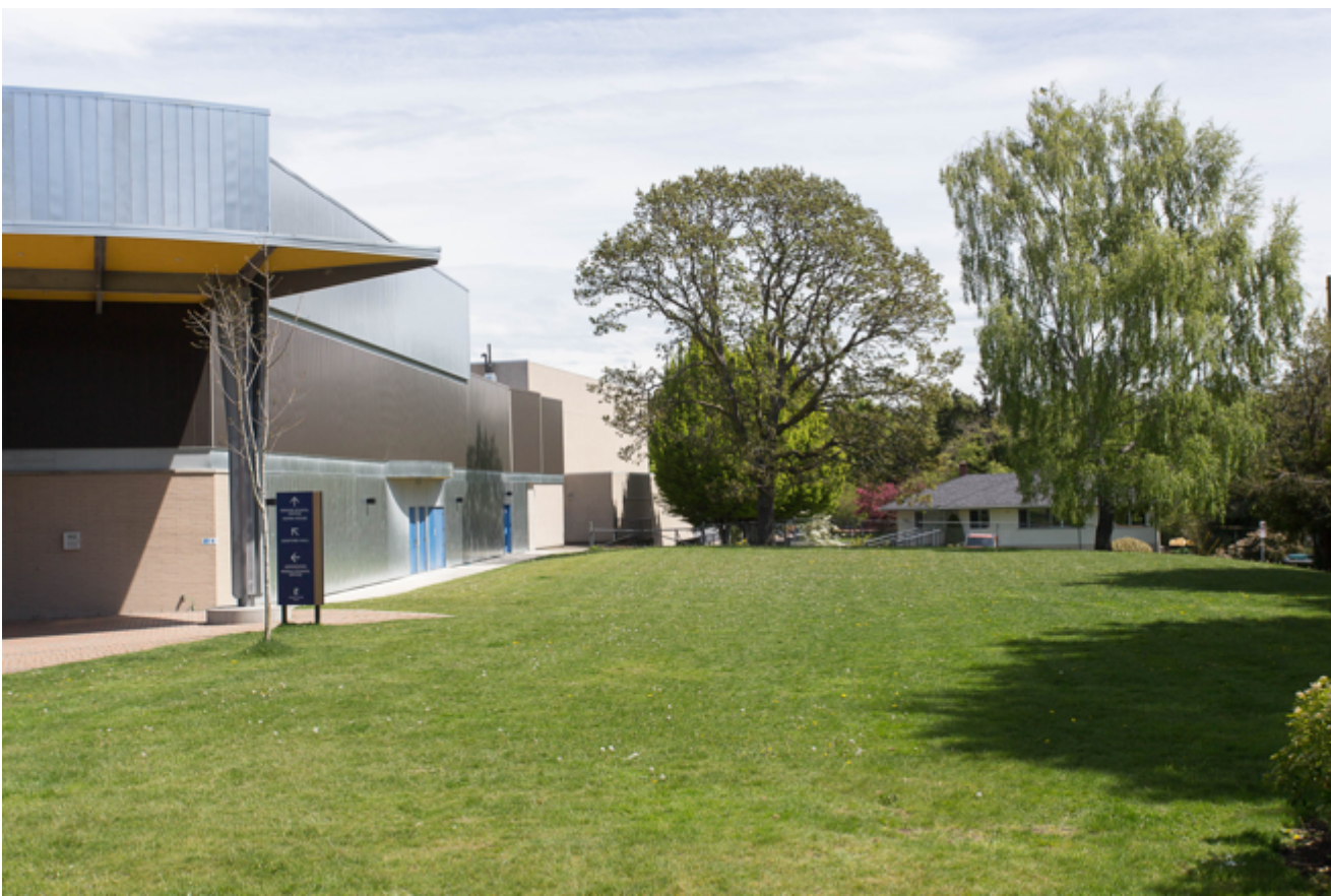
Views of site looking southeast
