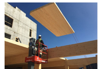
CLT floor panels at the Brock Commons Tall Wood House on the UBC Campus
