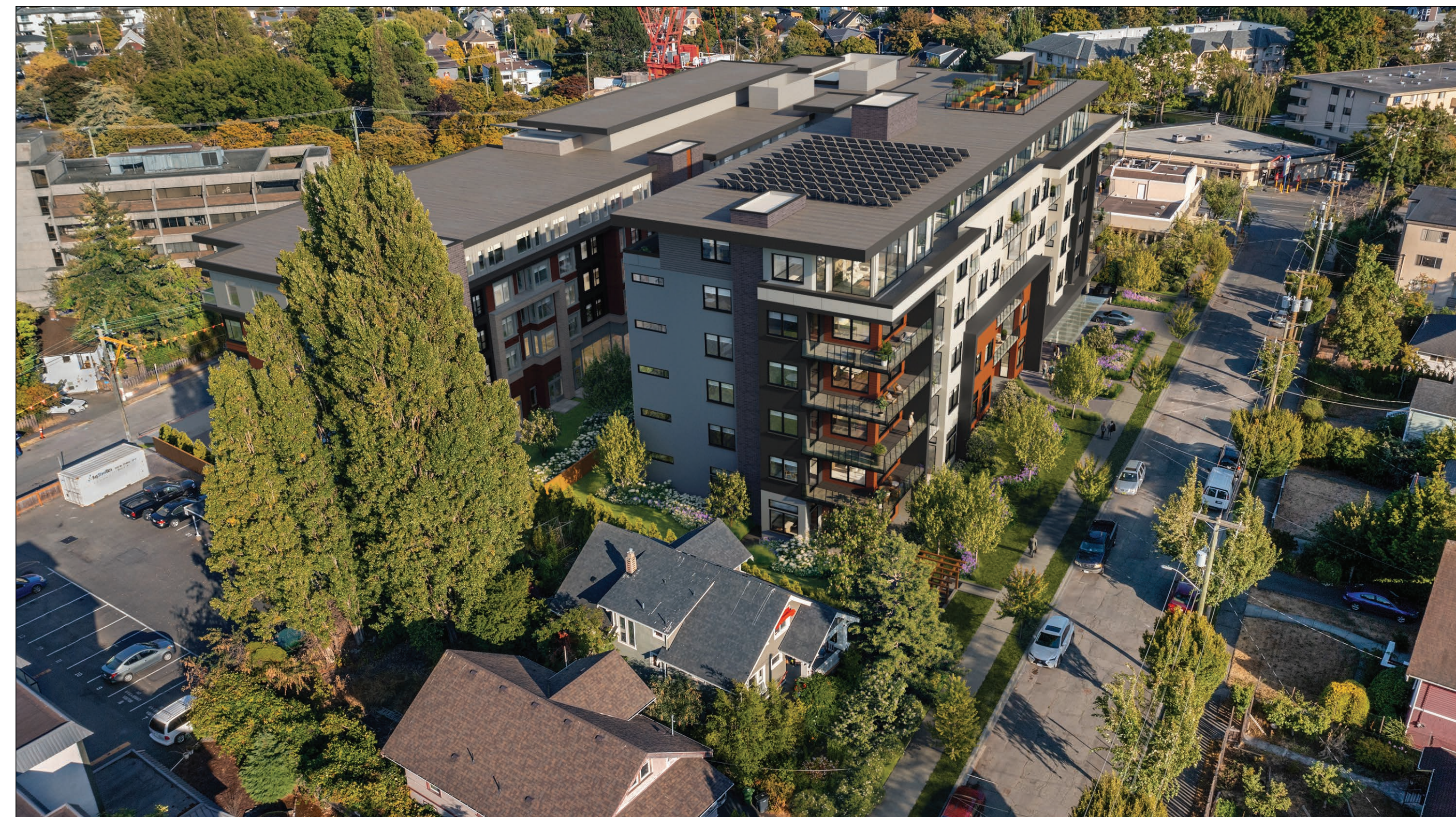
Aerial View - Looking South East from Ashgrove Street Phase 1 in Background
