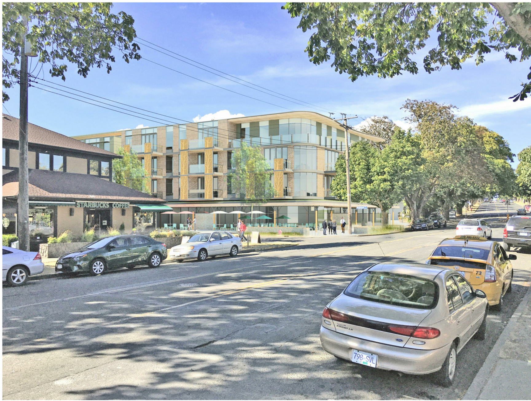
CORNER OF COOK STREET & PENDERGAST STREET
