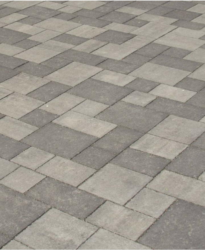
VEHICULAR PERMEABLE PAVING EXAMPLE
