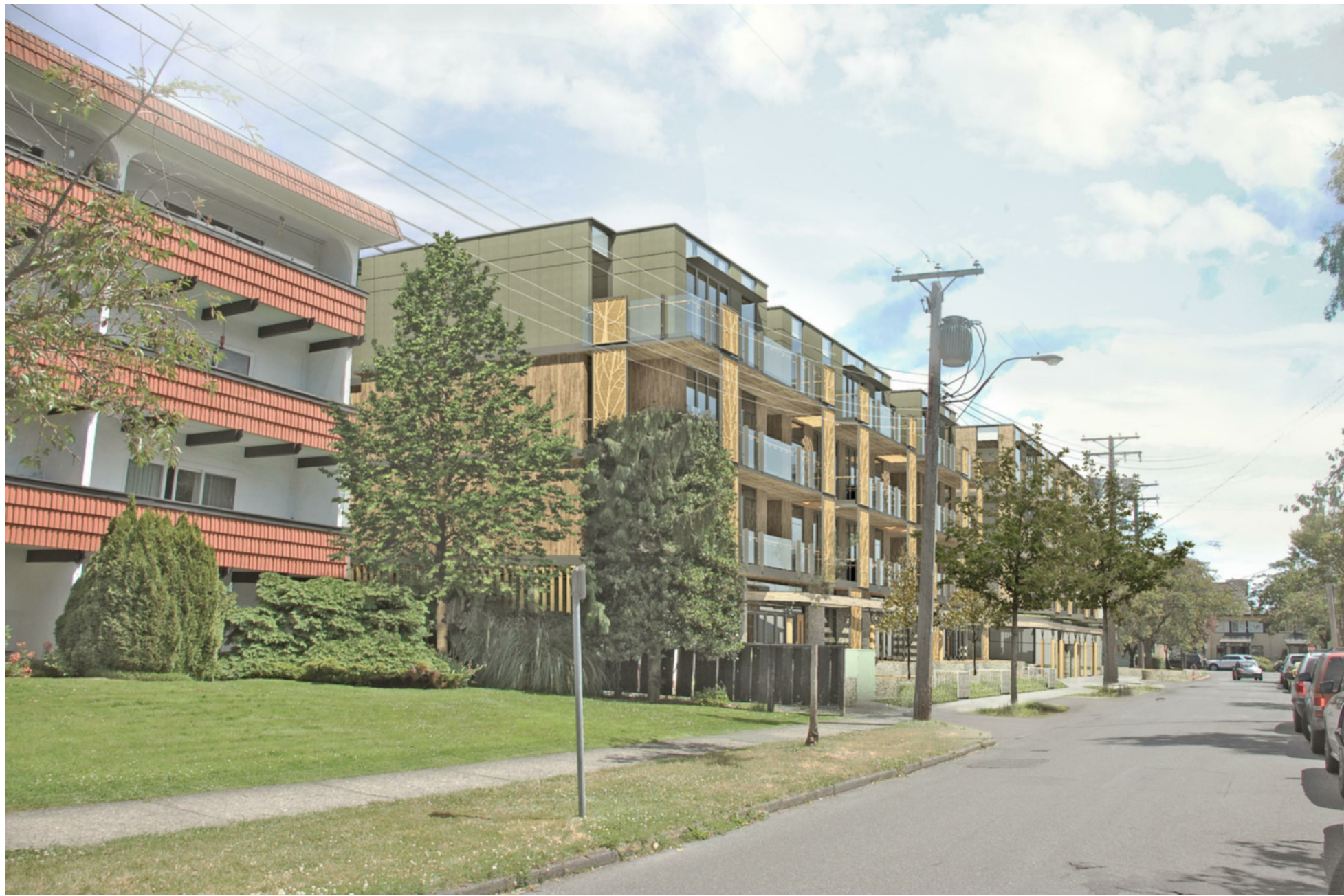
VIEW ALONG PENDERGAST STREET
