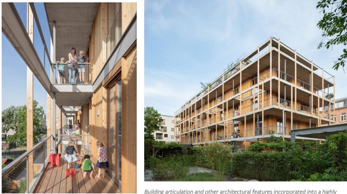
Thermally broken balconies and decks help create private and semi-private outdoor spaces for residents at a high-performance multi-family residential development.
