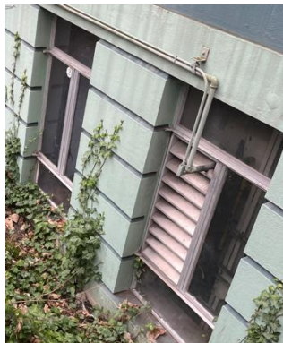
Window modifications to accommodate piping and conduit on lower north elevation.
