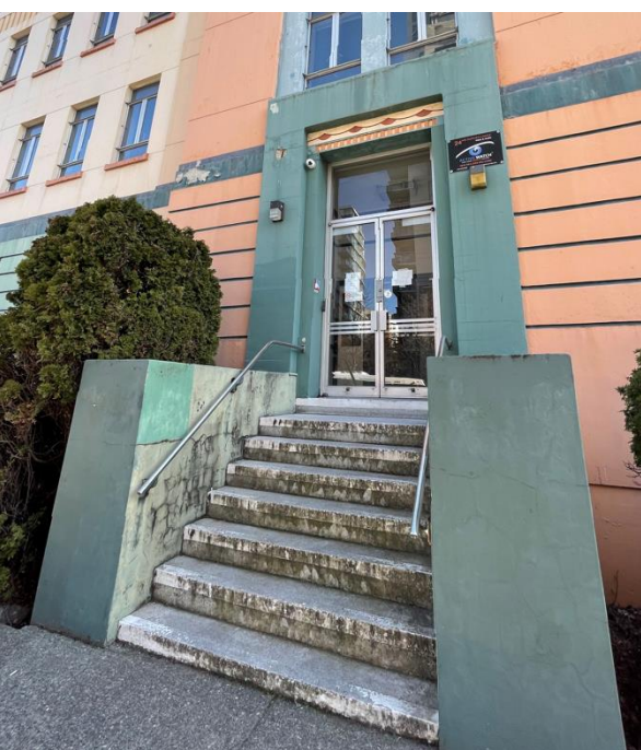
Surround around south entrance and closed stair retaining walls to be restored to their original appearance clad in marble.
