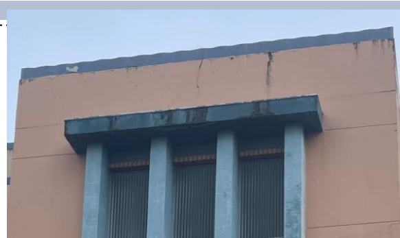
The upper projecting concrete canopy does not appear to be metal-clad along its fascia and overall deterioration of the canopy is not as severe as the lower canopy.
