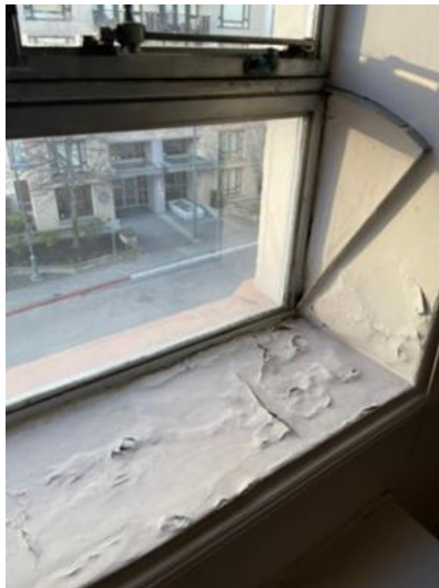
Deterioration of concrete sills and concrete surround throughout the building.
