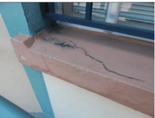
Cracks evident on window sill areas.
