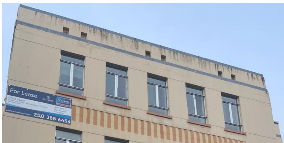
Stained wall surfaces clearly evident from the multi-colour palette applied in 1994.
