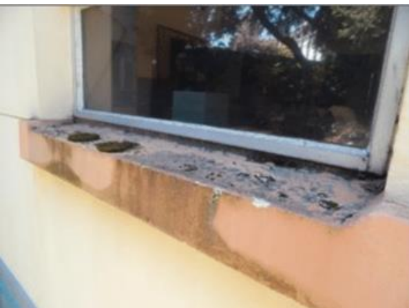
Organic accumulation and stains on window sills.
