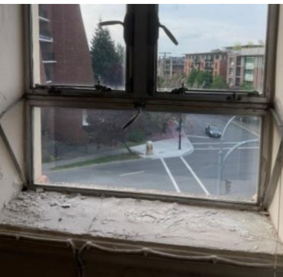
Deteriorated concrete sills, no evidence of waterproofing, and spalling paint a clear sign of moisture.
