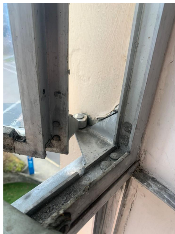
Deterioration of metal sections of the window frame.
