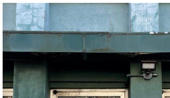
The lower projecting concrete canopy is metal-clad and appears far more deteriorated than the upper canopy, with corrosion, efflorescence on the concrete, loss of cladding material, and water ingress.
