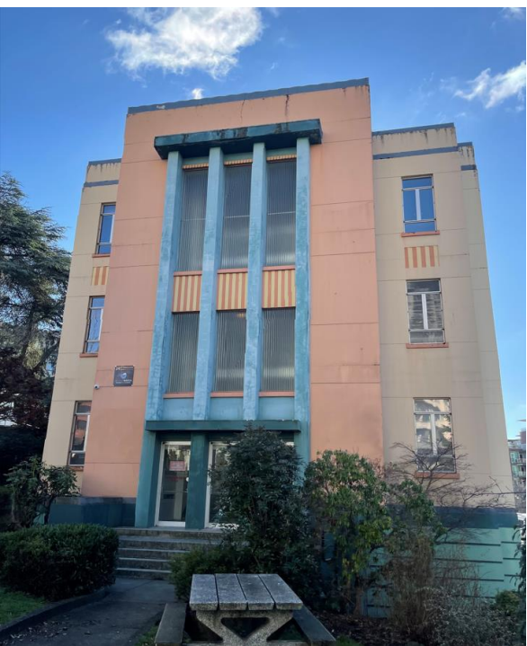
Four pilasters and closed stair retaining walls to be restored to their original appearance clad in marble.
