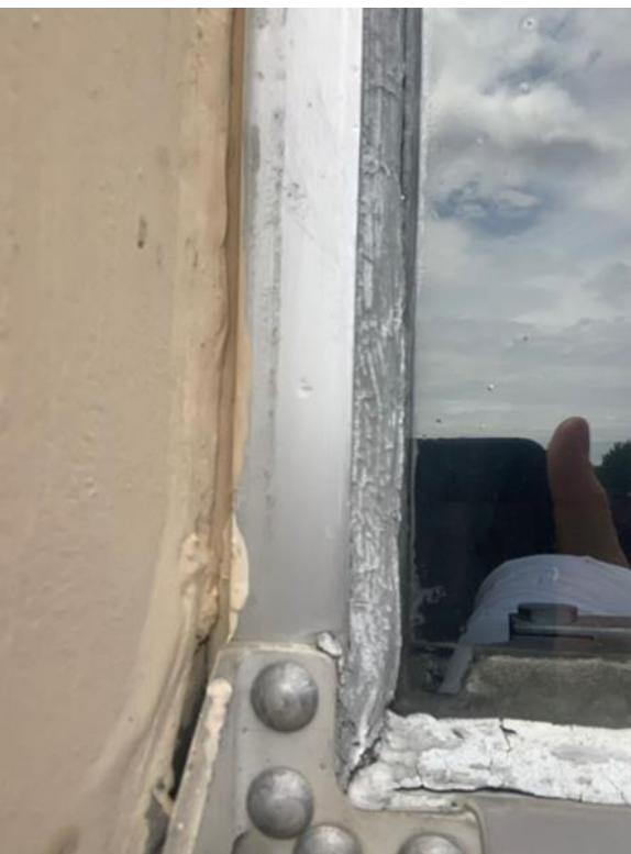
Deterioration of glazing compounds and lack of exterior perimeter caulking.
