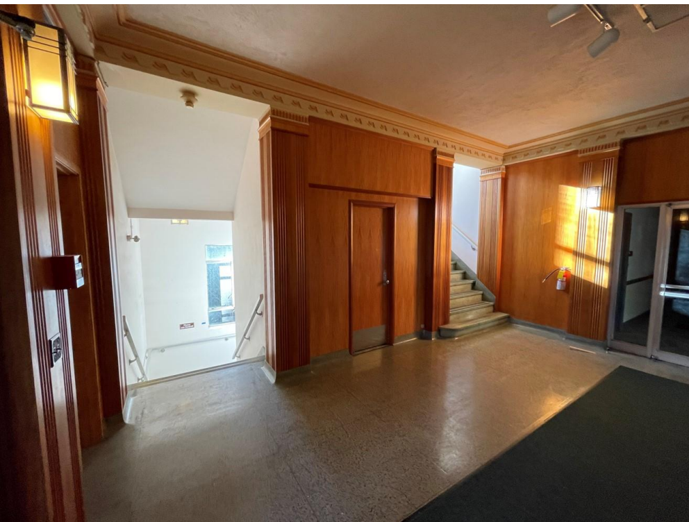
East side of interior lobby adjacent interior stair circulation connecting all floor levels. Note the flush wood panelling, fluted columns, and covings that provide a classical interpretation.
