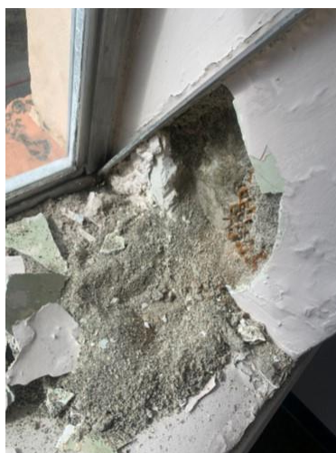
Deterioration of concrete, rusted metal mesh, and lack of a waterproof membrane at the sill and concrete surround.
