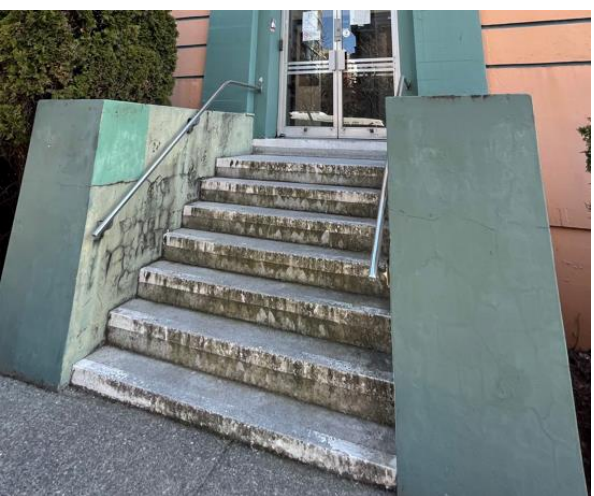
Cracks in closed stair retaining wall, as well as badly stained exterior stairs.
