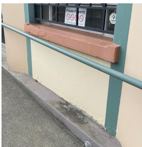
Organic accumulation and stains on base ledge.
