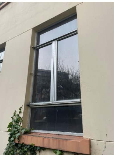
Above and below: Fixed and operable single glazed window units set within metal frames in punched openings.
