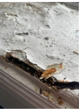
Deteriorated concrete sills, no evidence of waterproofing, and spalling paint a clear sign of moisture.
