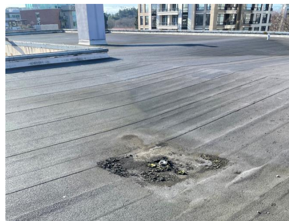
View of one of the roof drains in poor condition.
