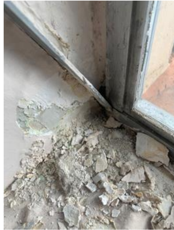
Loss of substrate integrity at several locations.
