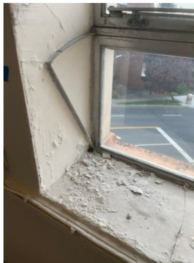
Deterioration of concrete sills and concrete surround throughout the building.
