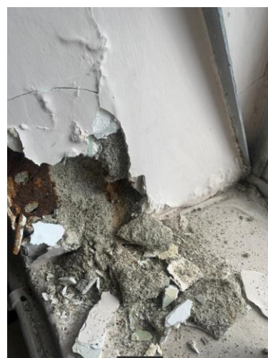
Deterioration of concrete, rusted metal mesh, and lack of a waterproof membrane at the sill and concrete surround.
