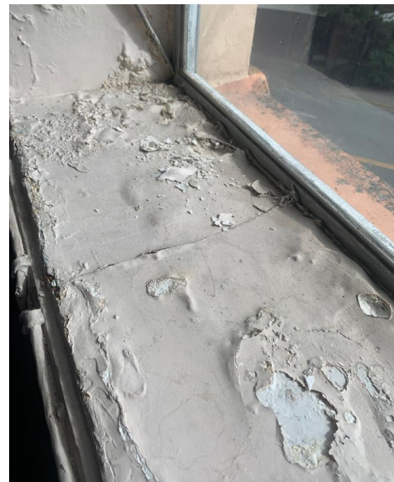
Paint bubbling and lifting from concrete surface. Lack of a waterproof membrane.
