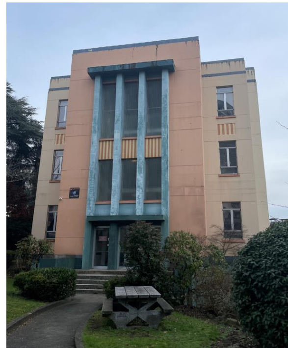
View of west elevation. Vertical pilasters and the closed stair retaining walls to be restored to original appearance clad in marble.
