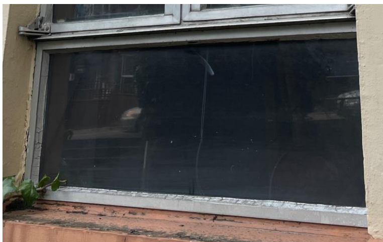
Deterioration of glazing compounds.
