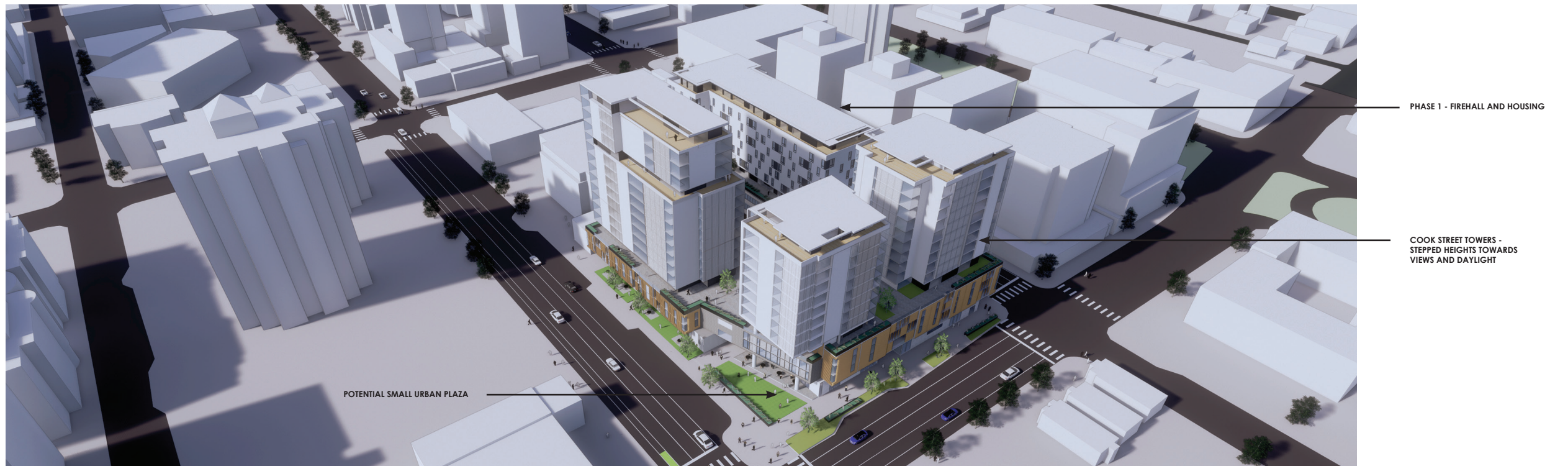
AERIAL VIEW OF POSSIBLE DEVELOPMENT
