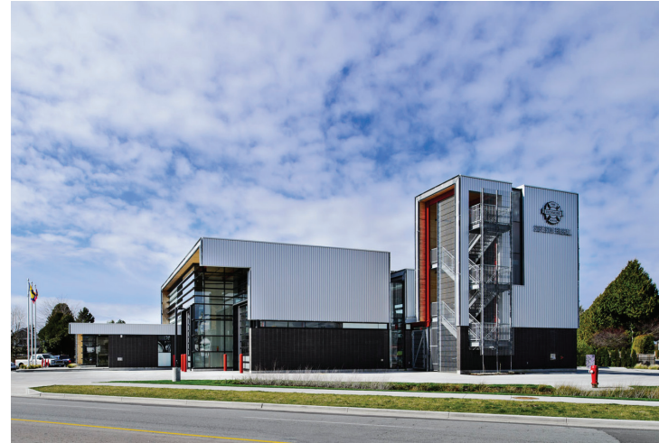
CONTEMPORARY FIREHALL STEVESTON FIREHALL 2 HCMA ARCHITECTURE AND DESIGN RICHMOND, BC
