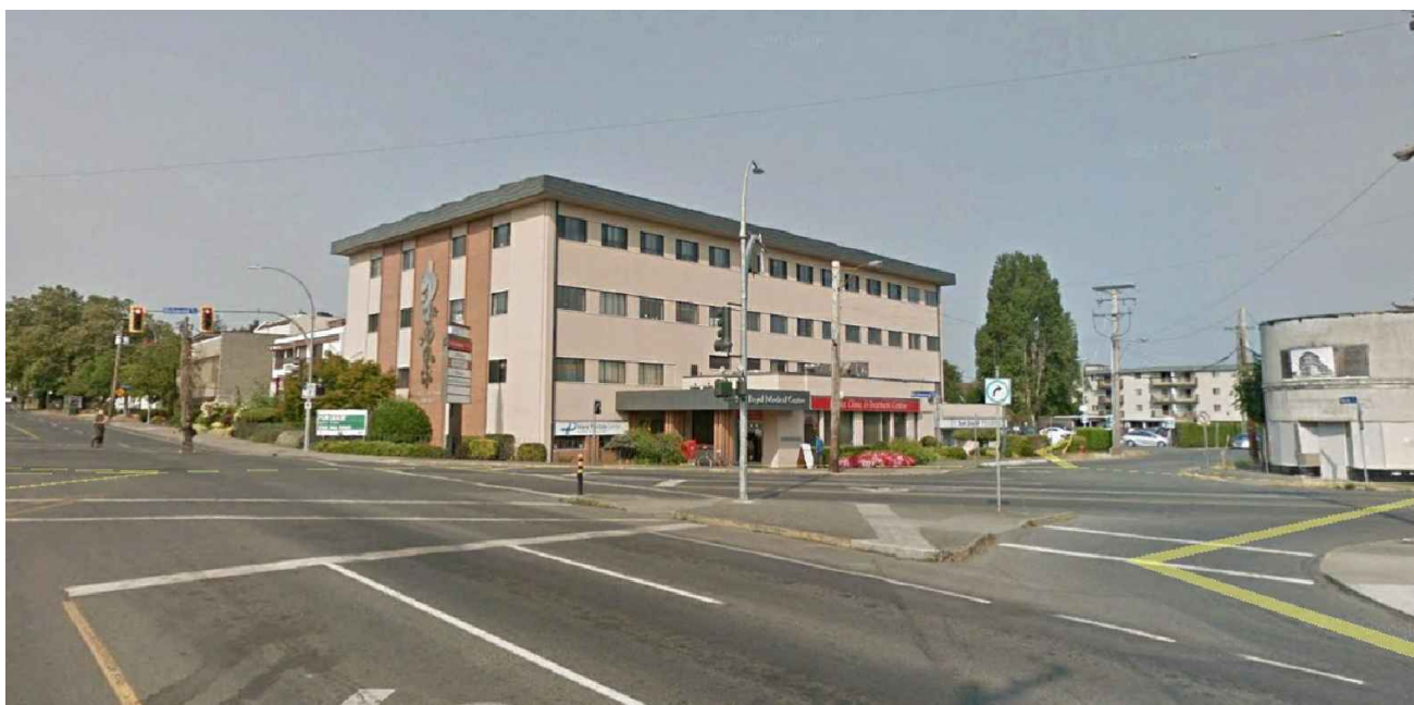
07 EXISTING SITE PHOTO FROM SOUTHEAST DP101 NTS
