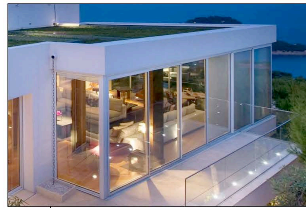
High-Performance aluminium and glass window-wall system
