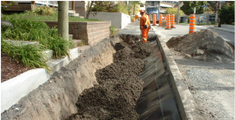
Structural soil installation
