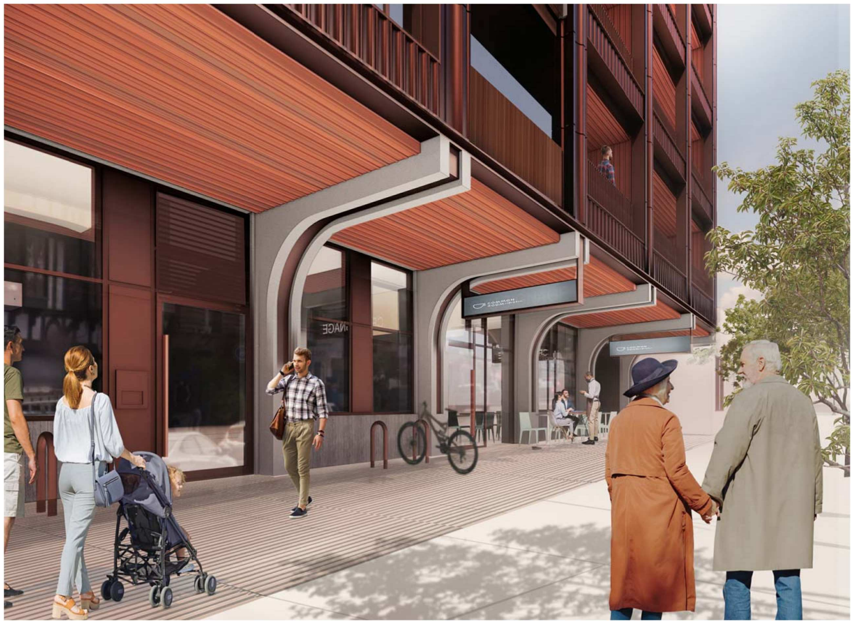
VIEW OF FORT STREET FRONTAGE
