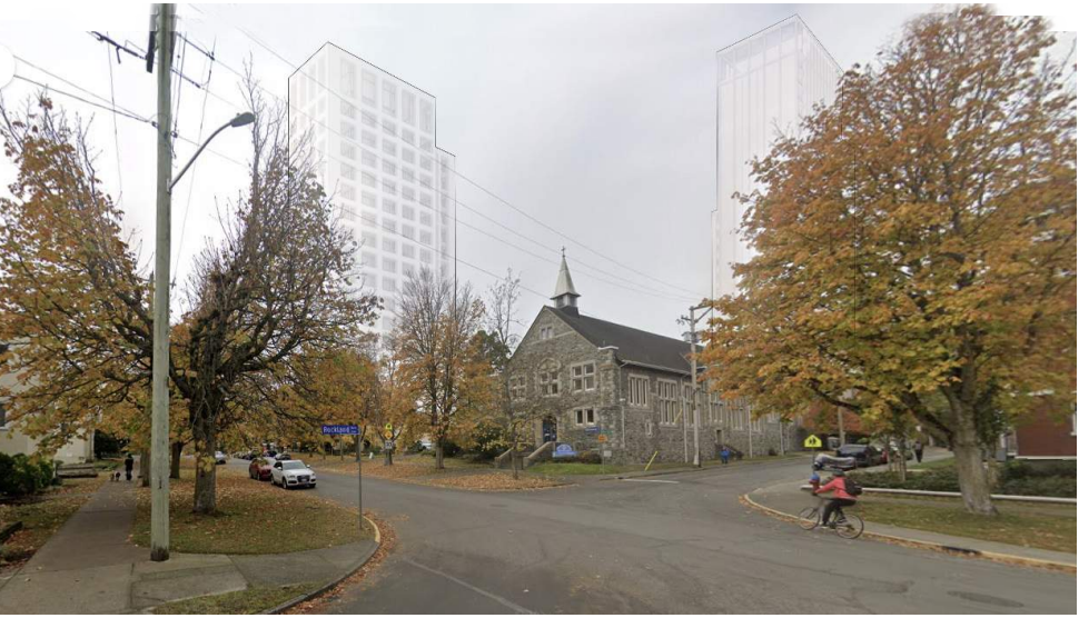
4. Rockland Avenue, looking south
