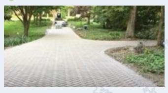
**Benefits:** Reduce runoff volume and improve water quality by infiltrating and treating stormwater while still providing a hard, drivable surface.
