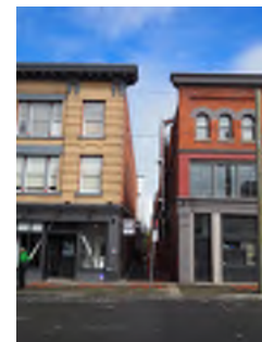
Image Reference # H6 Description: Break between buildings
