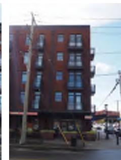
Image Reference # C7 Description: Adjacent Residential Building, Ironworks
