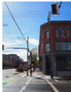
Image Reference # C1 Description: Commercial Building, Two Storey Residential
