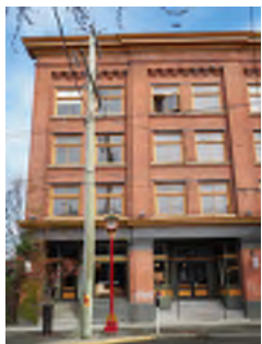
Image Reference # H4 Description: Adjacent Existing Building, Biggestuff Building (Historical)
