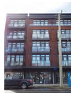
Image Reference # C6 Description: Adjacent Residential Building, Ironworks
