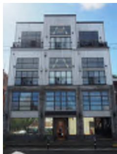
Image Reference # C3 Description: Adjacent Commercial & Residential Building
