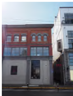
Image Reference # C2 Description: Adjacent Commercial Building, Two Storey Residential
