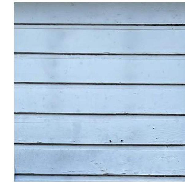
S1 EXISTING CHANNEL RUSTIC SIDING
