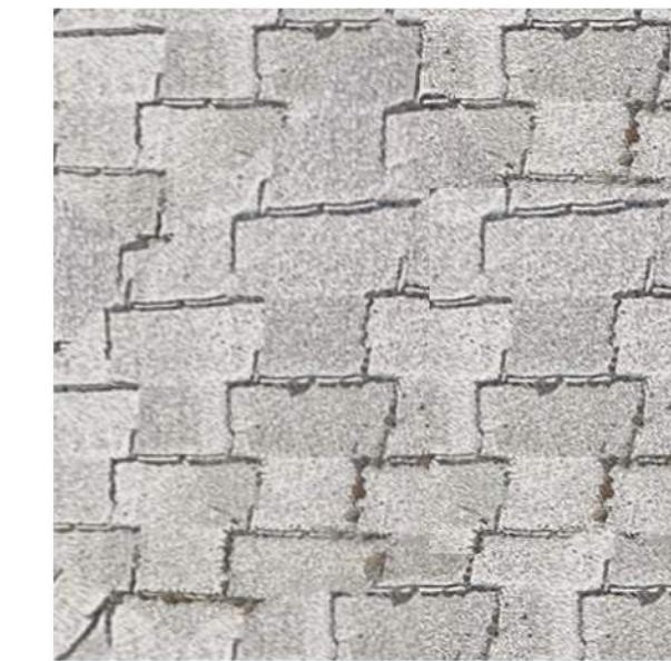
R1 EXISTING ROOF SHINGLES
