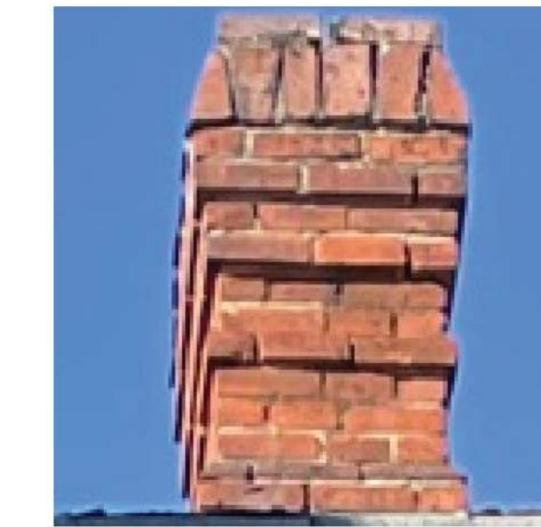
B1 EXISTING BRICK
