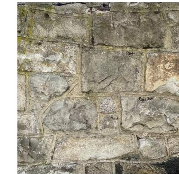
F2 EXISTING FENCING WALL
