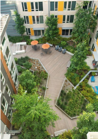
Landscaped courtyards (Eleanor Apts, Seattle by Hewitt)
