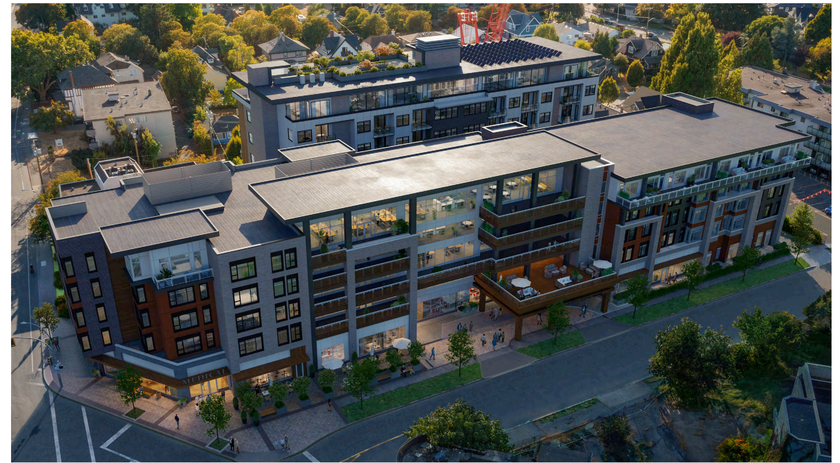
Aerial View - Looking South West from Richmond Road Phase 1 in Foreground
