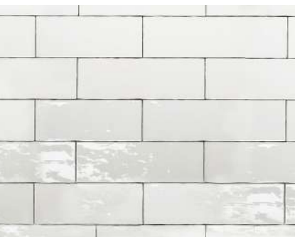
EXISTING WHITE GLAZED BRICK
