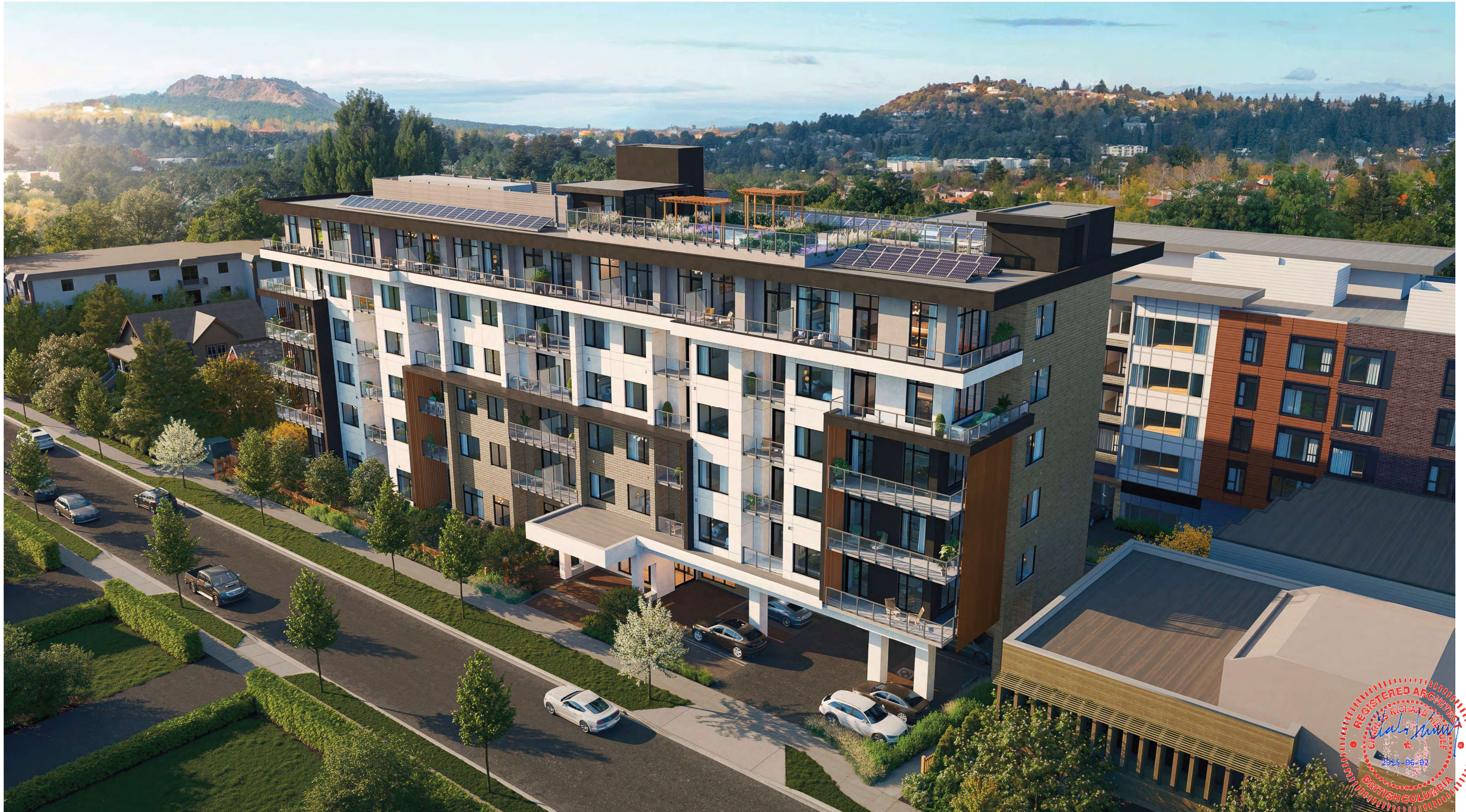
Aerial View - Looking NE above Ashgrove Street
