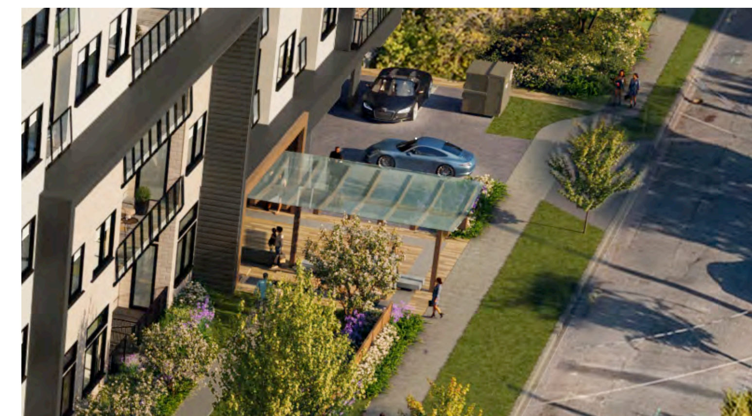
Main Entrance Plaza and Canopy
