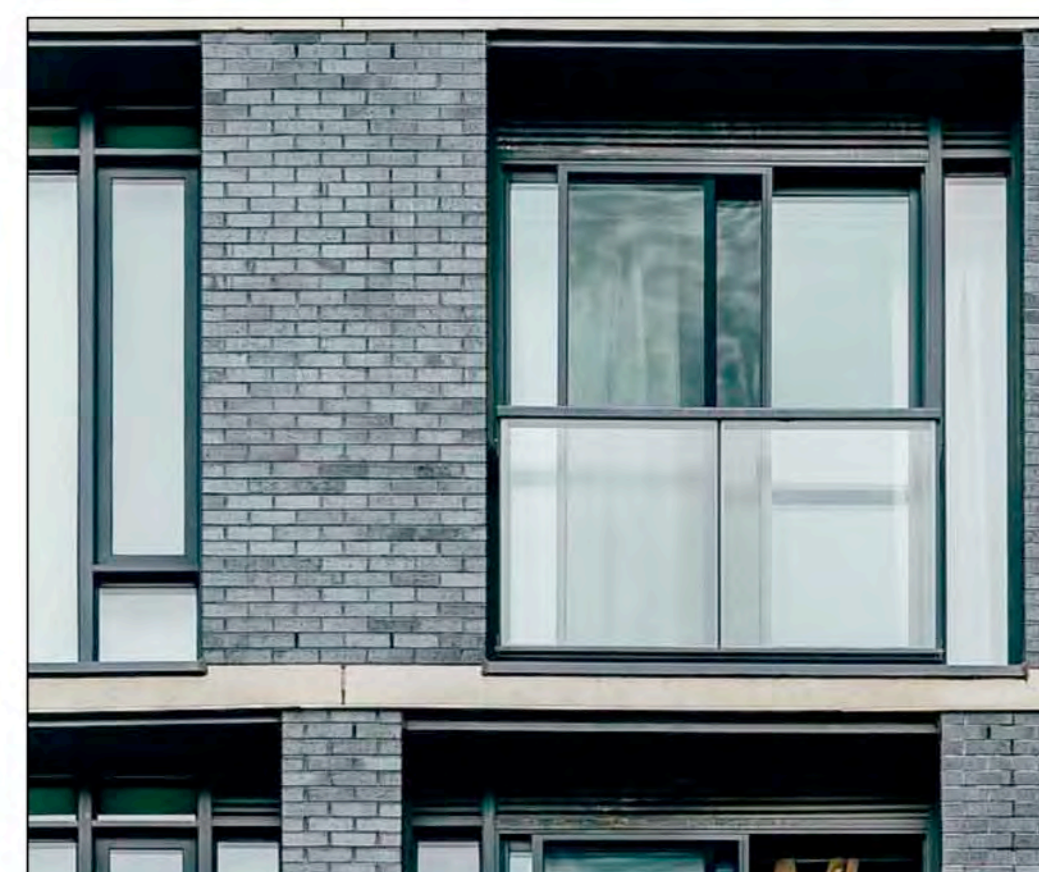
High-Performance vinyl windows with coloured frames
