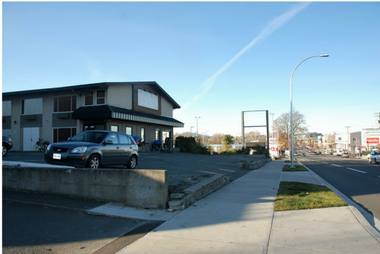
07. Site from Douglas St- looking north
