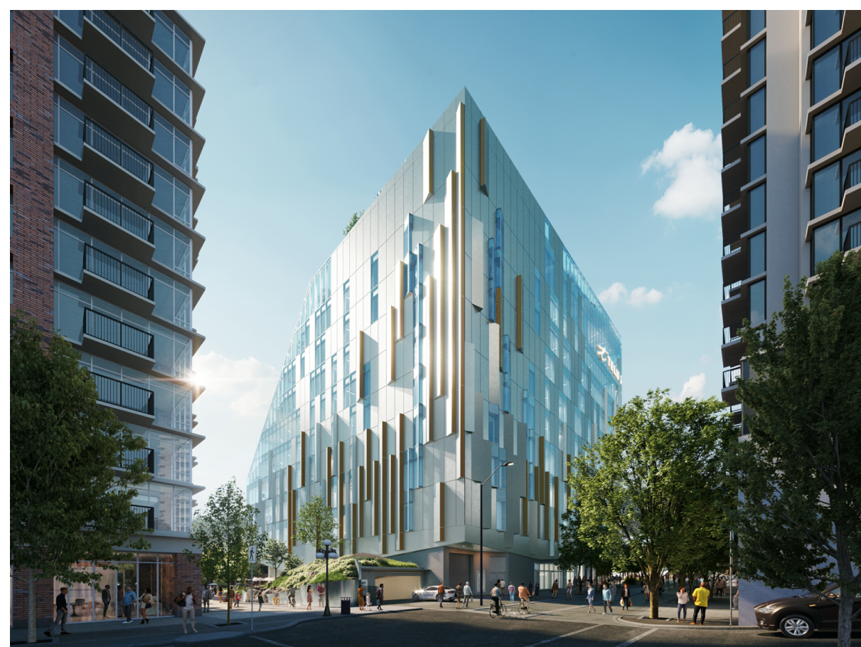
View from Humboldt and Penwill intersection
