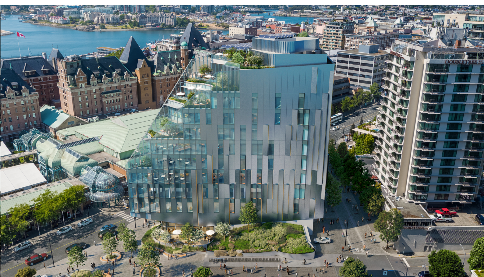
View of the Penwill facade
