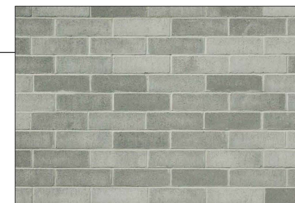
Smooth face masonry cladding
