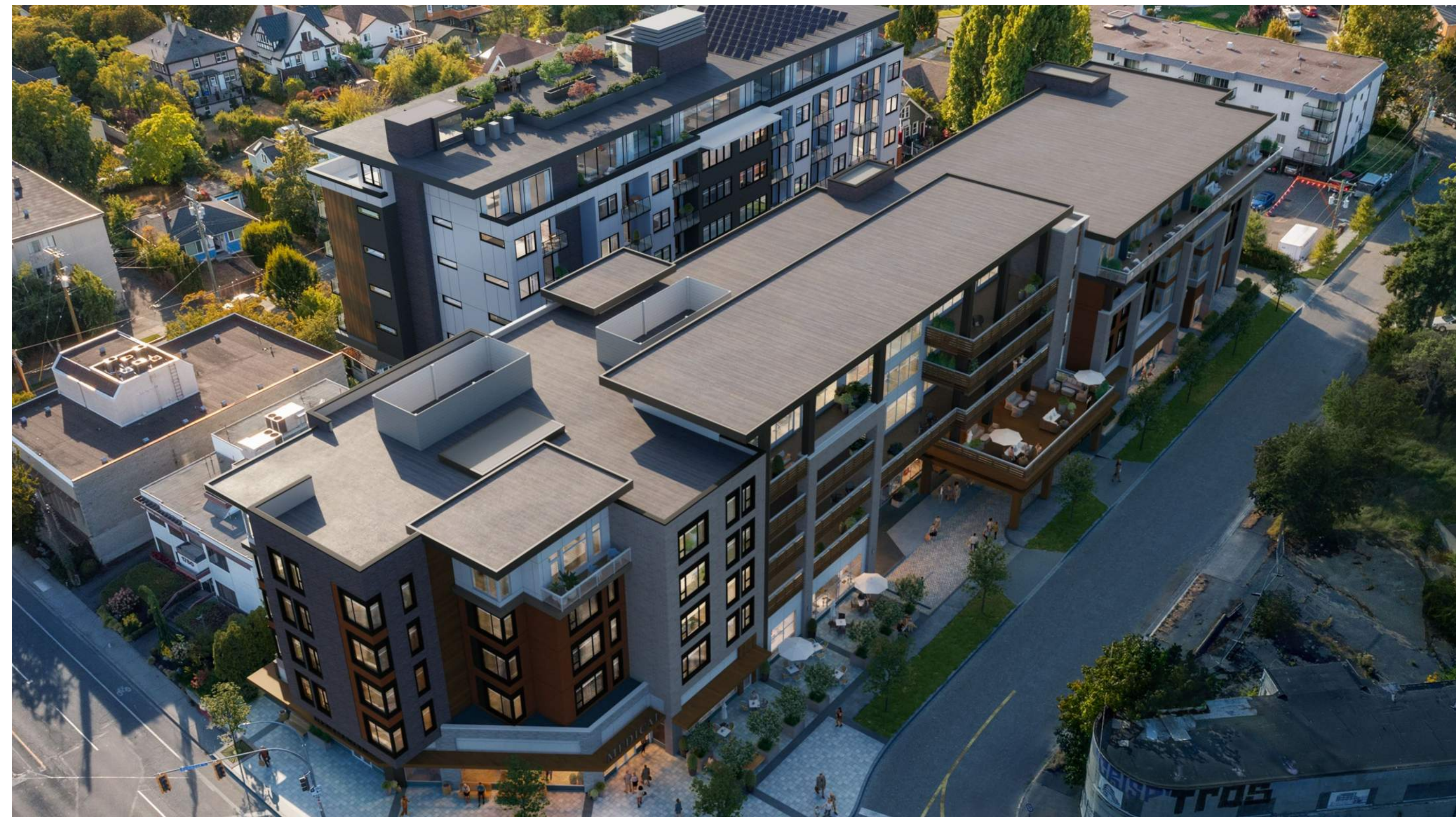
Aerial View - Looking West from Richmond Road Phase 1 in Foreground
