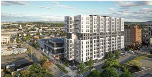
2615-2629 Douglas St. D'Ambrosio Architecture + Urbanism
