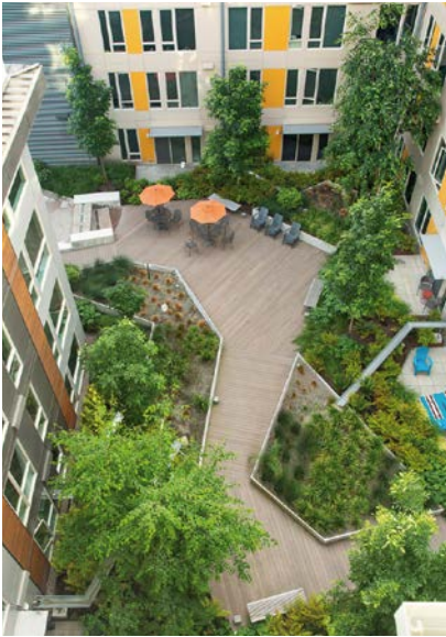
Landscaped courtyards (Eleanor Apts, Seattle by Hewitt)
