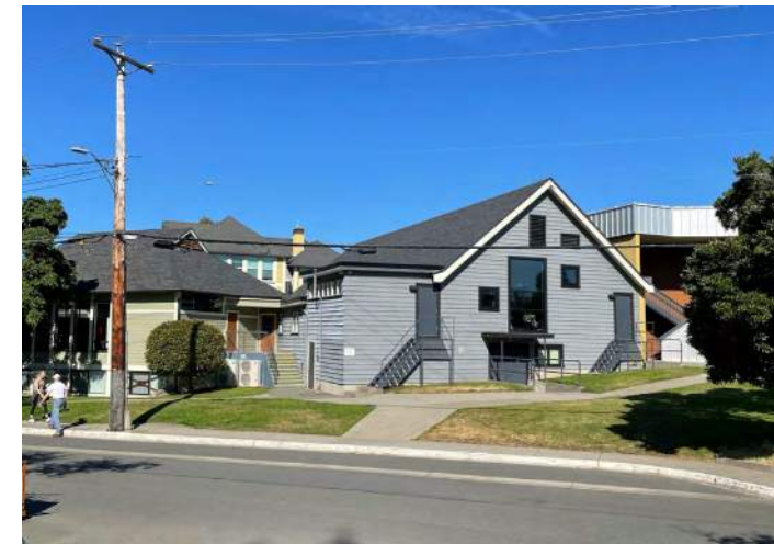
7: NORTH EAST CORNER OF SITE
